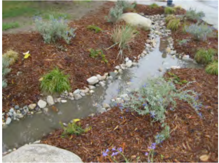
Figure 5: Water filled vegetated bioswale
