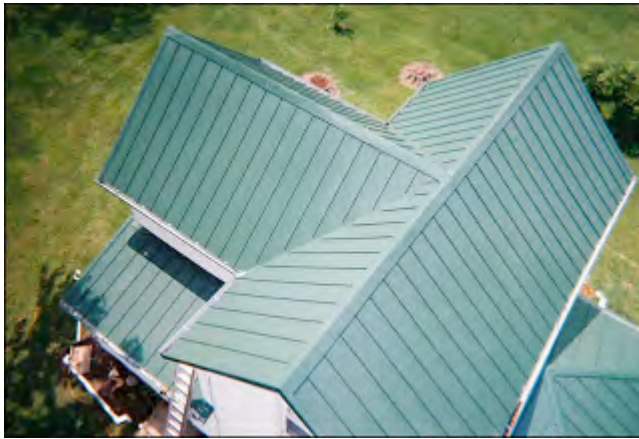
Figure 7: A Typical Residential Roof
