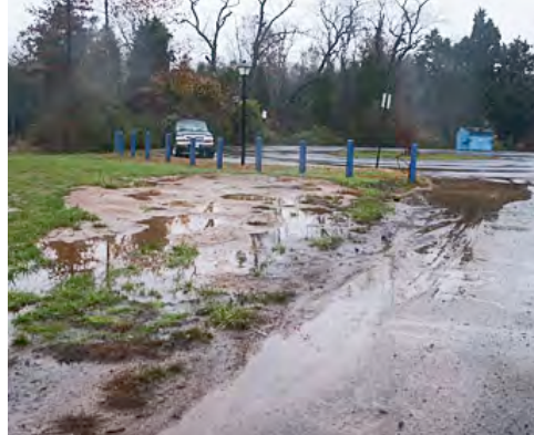
Figure 12: Displaced rain water runoff
