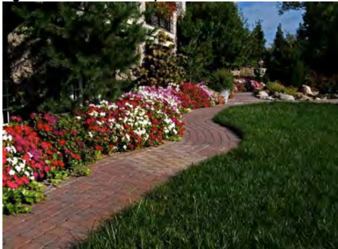
Figure 5: Permeable Clay Brick Pavements
