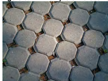
Figure 6: An Example of Porous Paving
